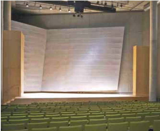
College of Art auditorium using a combination of reflective and 2" absorptive panels finished in Metallo.
