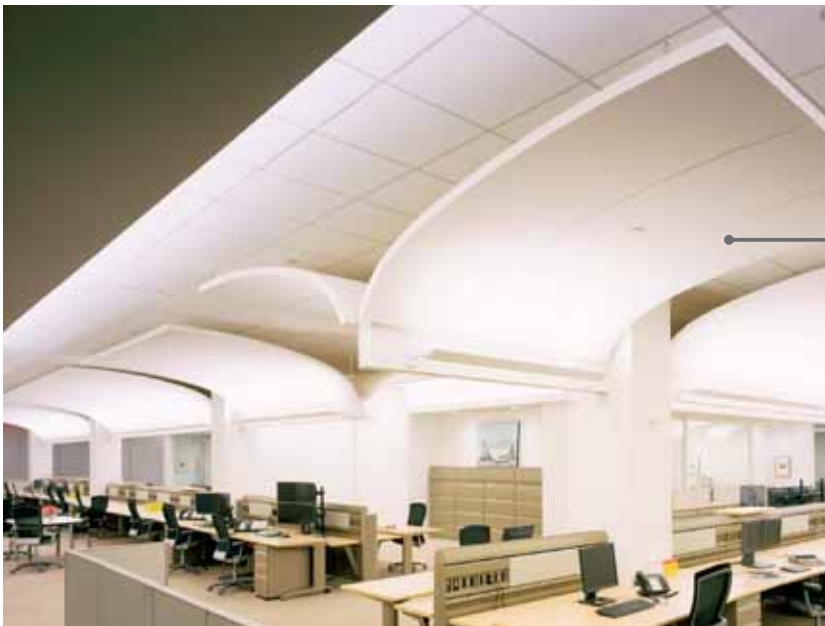
The irregular curvature of the 2-1/4 inch thick panels provides a unique architectural element and exceptional acoustic performance for the renovated offices of this financial management company.
