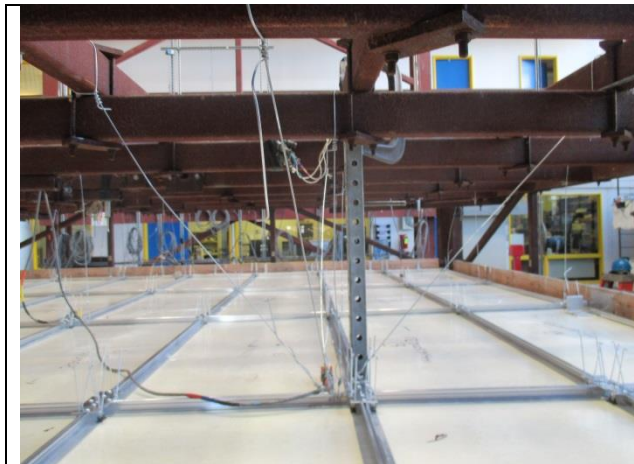
Photo 3: Four Way Splay Wires and Compression Post
