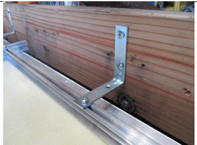
Photo 4: Clip Angle at Fixed Sides
